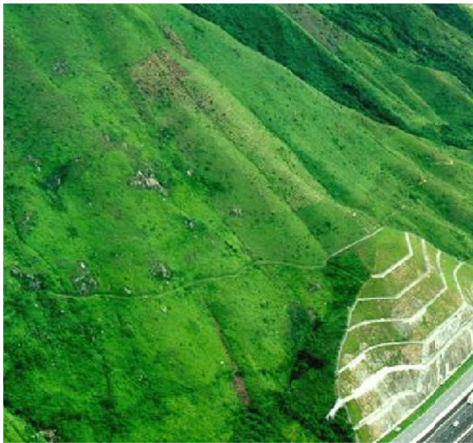
Fig 3B: This cut slope at the road level has very large upslope catchments which are prone to excessive infiltration. Adequate mitigations against signs of excessive infiltration plus instrumentation should be provided to mitigate against landslide.
